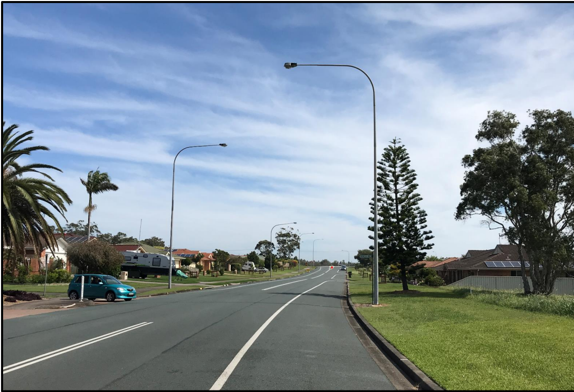
Photo 1 – View south along The Southern Parkway adjacent to the subject site. Note footway on left hand side of photo.
